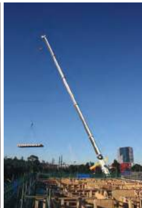
Clockwise from above: Services and penetrations form part of the Demonstration Model; lifting Tilling floor cassettes into place at The Green; SmartJoist and TecBeam formed the floor joists and roof for the four-storey DHHS Preston Renewal Stage 1 in Melbourne.
