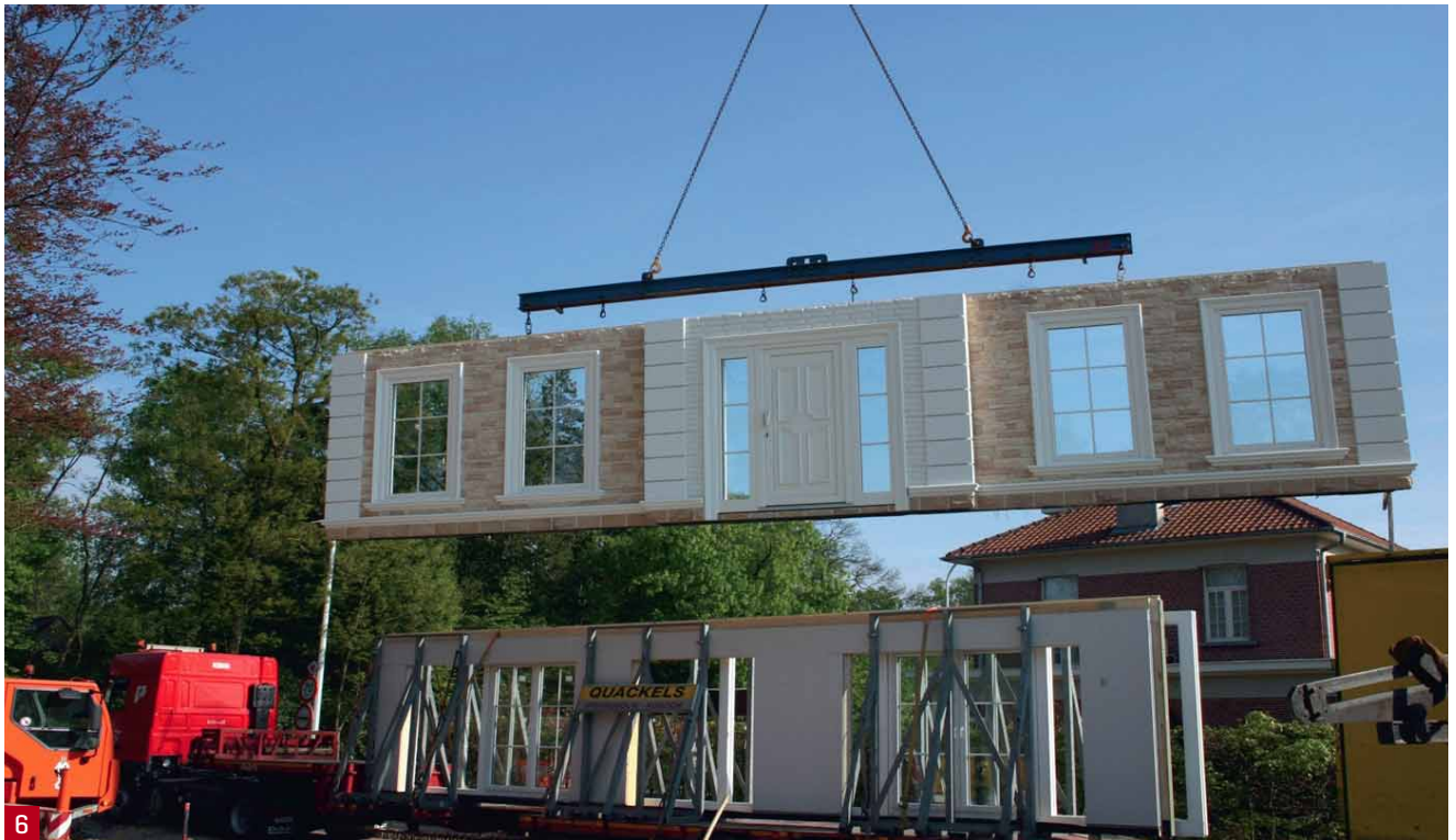
IMAGE 6: Completely prefabricated wall panel in Europe.
